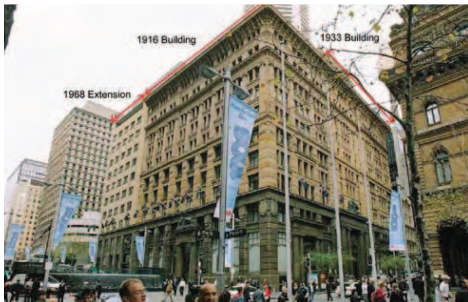
Figure 6 – North-west corner, looking south along Pitt Street best showing the 1916-1933 component of the building and the 1968 extension
