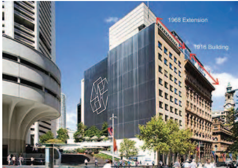
Figure 8 – North-east alignment of the building illustrating the context of the buildings on the site and the 3 storey plant room fronting Martin Place
