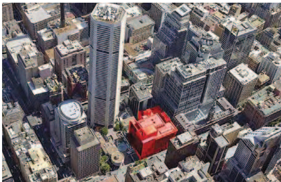
Figure 2 – Site context with the existing building on the site highlighted in red
